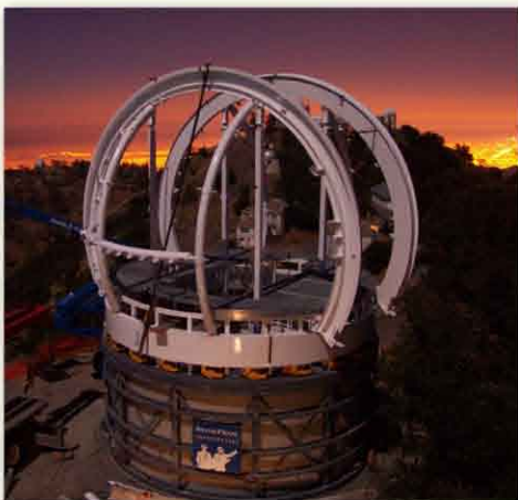
APF Under Construction
