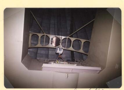
Out had most be used for litting mirror from lelescope, Use a length of chain from floor payling of the between hook & athrex chains. Lont use the extra hook on the long chain. Chain lengths 2-45" 1-77"
