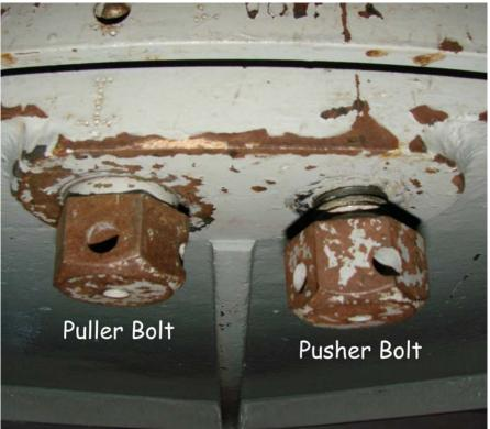
This is an image of the push pull bolts used for aligning and removing the mirror cell. When removing the cell **NEVER!!** move the pusher screws. Moving the pusher screws will misalign the mirror.
