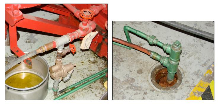
The hose hooks to the Kinney pump just above the pressure regulator and flows out into the drain in the floor. Remove the pipe plug in the drain assembly to see that water is really flowing from the two pipes then replace the pipe plug.
