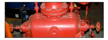
Turn on the pump by pushing the start button then close the two back pressure relief valves shown in the picture above. Close both right and left valves by turning them clockwise.
