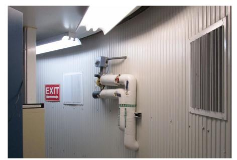
The valve for FCU 1 is mounted on the wall of the dome in between the two air vents (see below.) Turn it to the on position, the opposite of the picture below.
