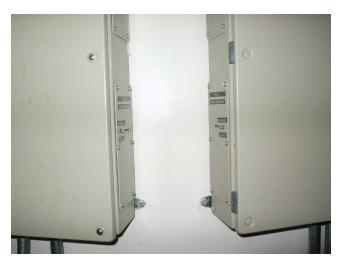
Each has a switch mounted on the side which will turn on the fans. The Fuse Cabinets for Fan Controller Units 1 and 2, showing the switches to turn the fans can be seen to the left.
