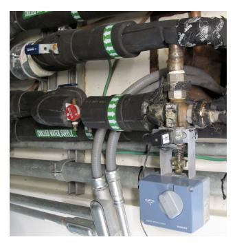
The valve for FCU 2 is to the left of the fuse box and is mounted sideways. Turn it to the full on position. Those valve knobs have to be pushed in while turning.
